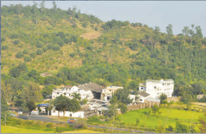
HEX - BCA factory at Vapi, Gujarat
