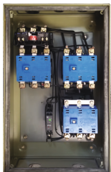
Interior View of ML FASD
