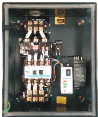
Interior View of MU-G10W DOL
